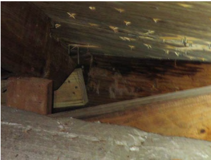
Rust drain pan
