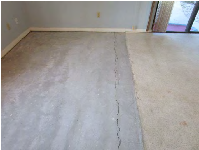
Cracking floor
