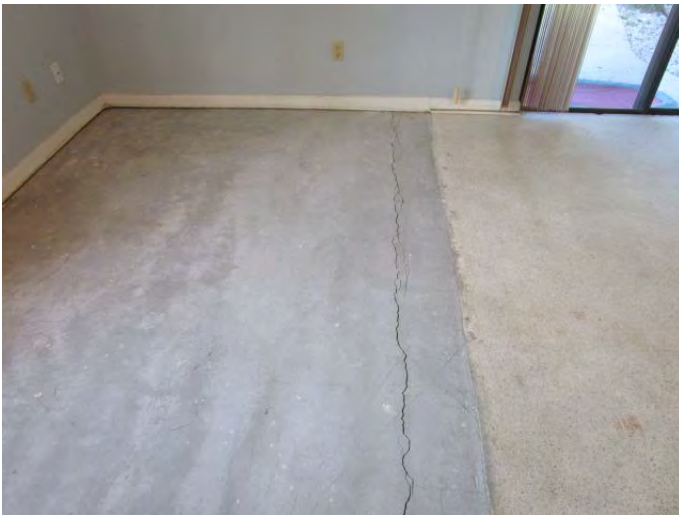
Cracking floor
